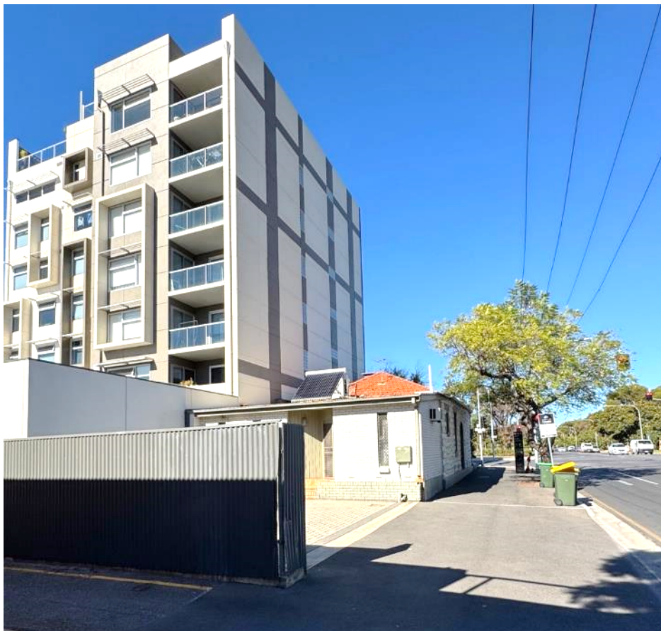
Photo 3.5 – Looking south from eastern side of Morphett Street
