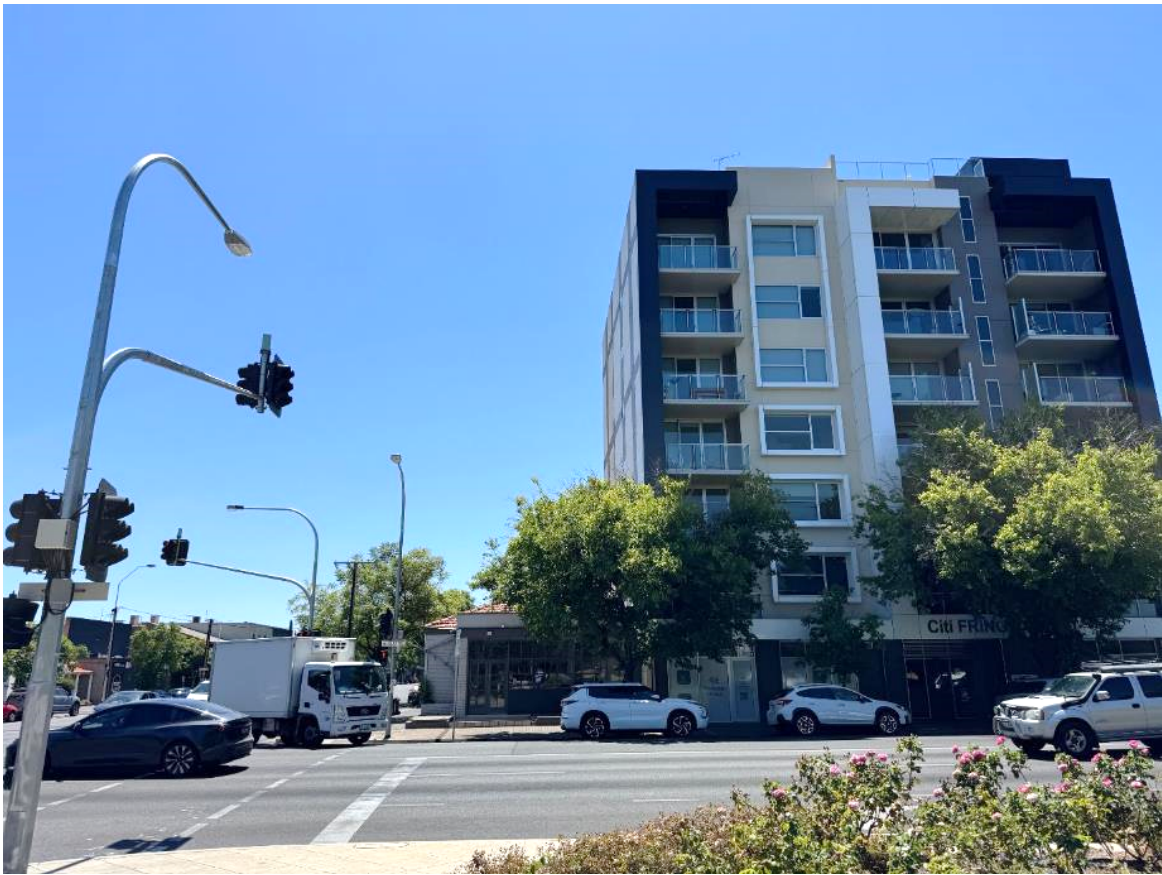
Photo 3.1 – View of subject and adjacent site looking north
